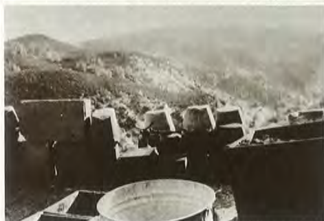
Above: In the early days, Stauffer refined crude sulfur blocks on site at a number of its own small mines in California. Below: most of Stauffer's sulfur comes from the mines in the Texas Gulf Coast area where the sulfur is pumped out of the ground in molten form by the Frasch sulfur recovery process.
